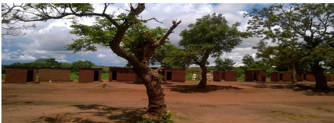
b. Traditional latrines without a hand washing facility nearby (Source: In-depth study 2016)
